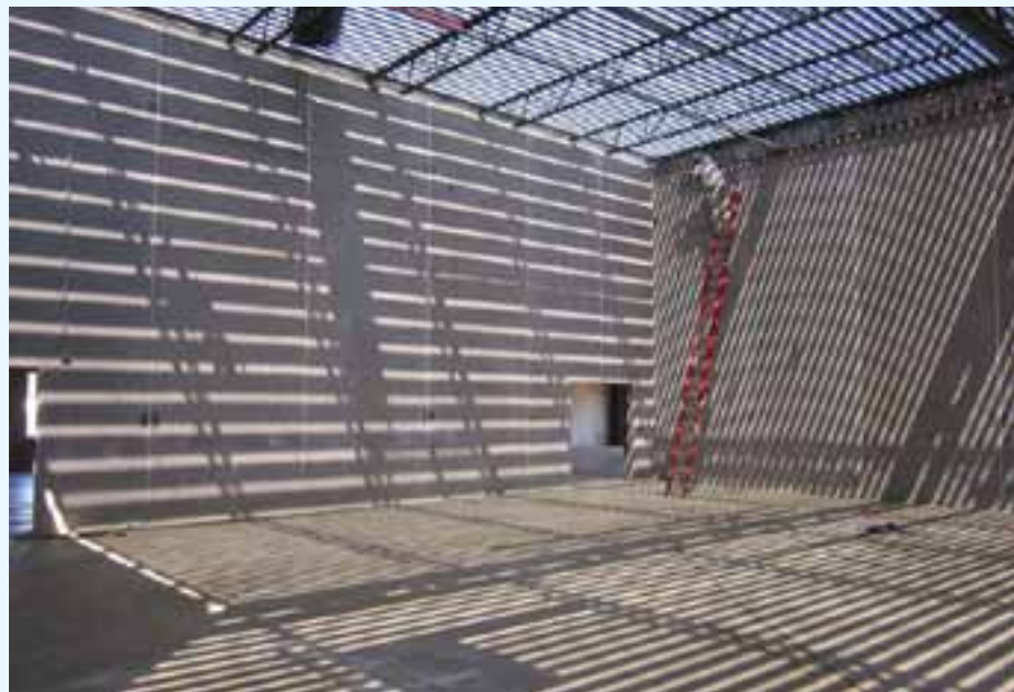
Construction crews are busily erecting a new 37,000-square-foot permanent school building for Imagine Andrews.
